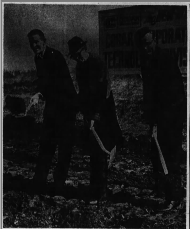
COGAR GROUNDBREAKING ceremonies were conducted Thursday at the 64-acre site in the Town of Wappinger. Left to right are George Cogar, Supervisor Louis Diehl and Robert Markle, manager of the local division.
